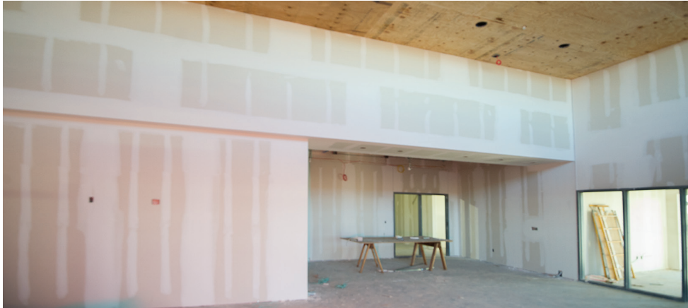
LOBBY INTERIOR ON JAN. 16, 2015
